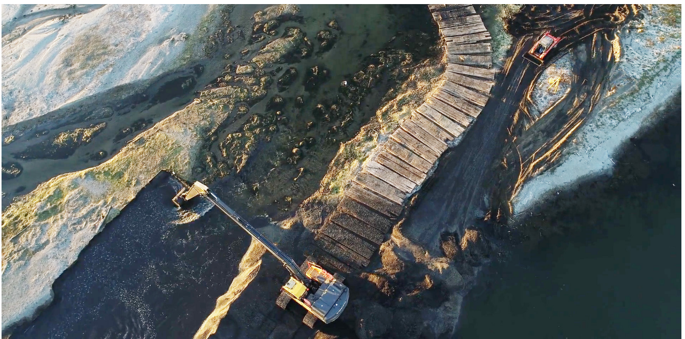
Figure B-8: Sediment Removal Project at Lake Poinsett Outlet
