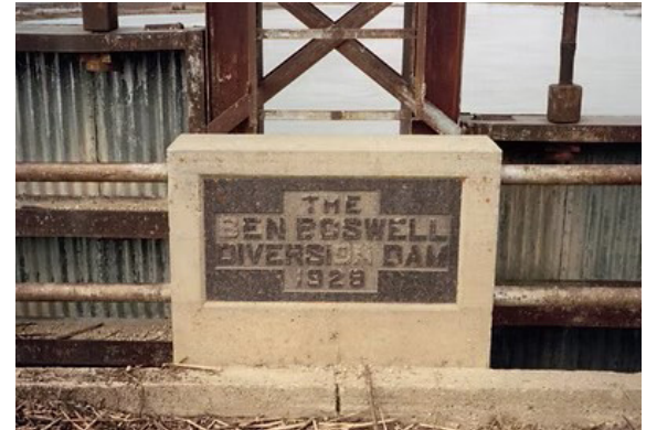
Figure B-1: Boswell Diversion Structure
